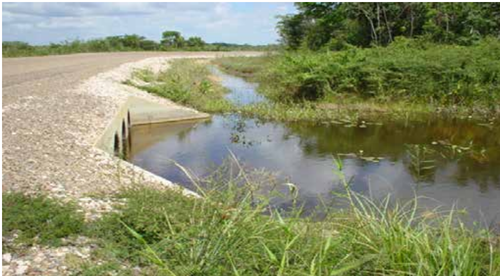
Figure 21. Maintaining the Flow of Water
