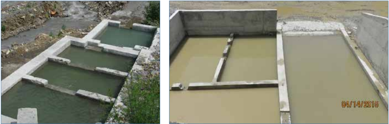
Figure 12. Multiple Stage Sedimentation Tank
