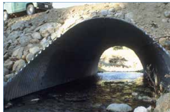
Proper Placement of Culvert
