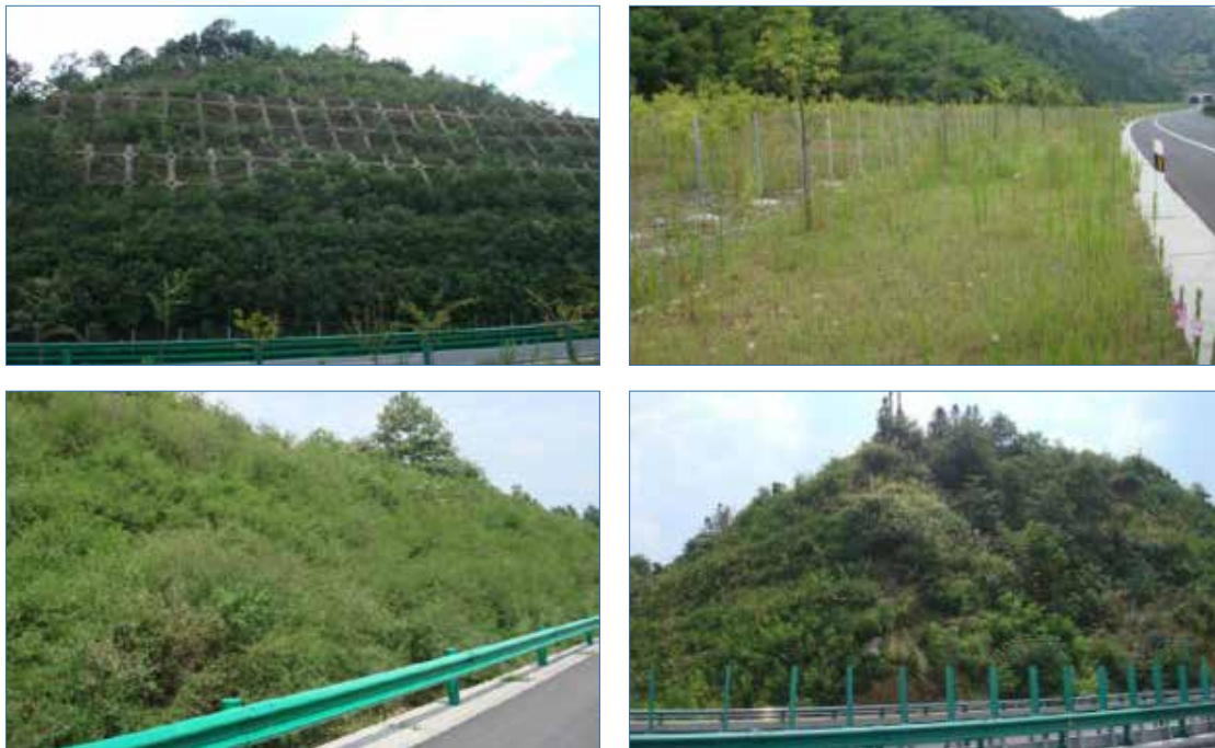
Figure 27. Slope Stabilization, Landscaping, Reforestation
