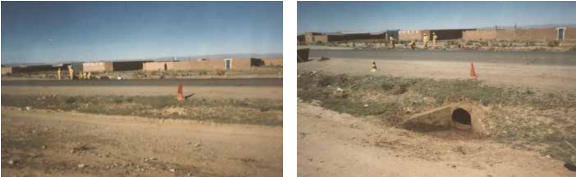
Culvert before and after maintenance activities
