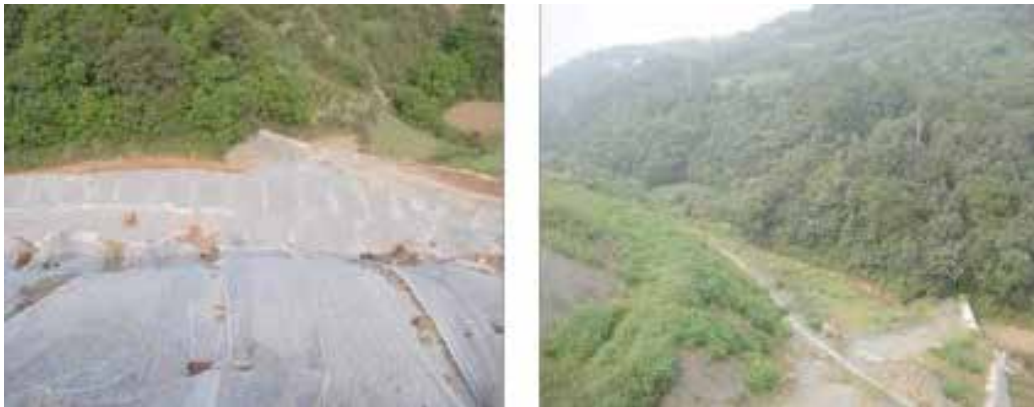
Figure 15. Restoration of Borrow Areas
