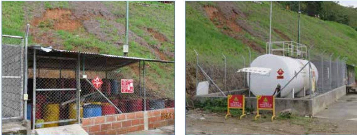
Figure 14. Proper Management of Chemicals
