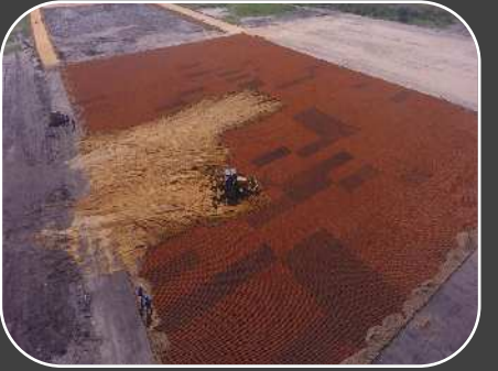
Geocells being filled with sand/saibro (laterite) mix
