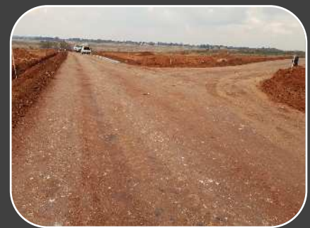
SoilTech Mk. III Polymer Stabilized
